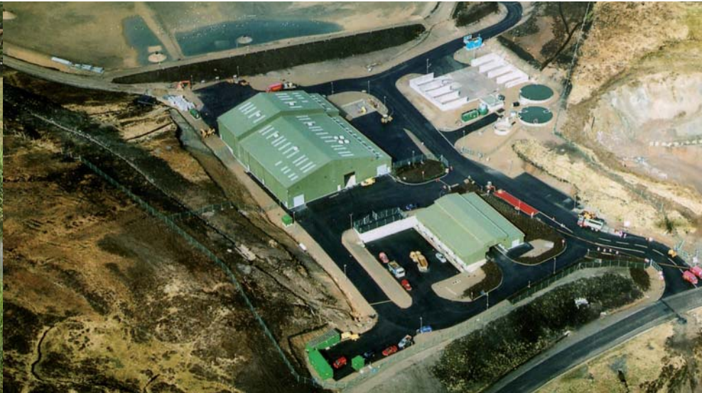
Gramista landfill leachate treatment facility.
