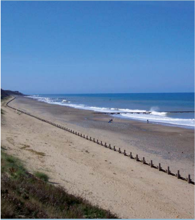
We evaluated the impact of a gas pipeline installation on the foreshore at Bacton, England.
