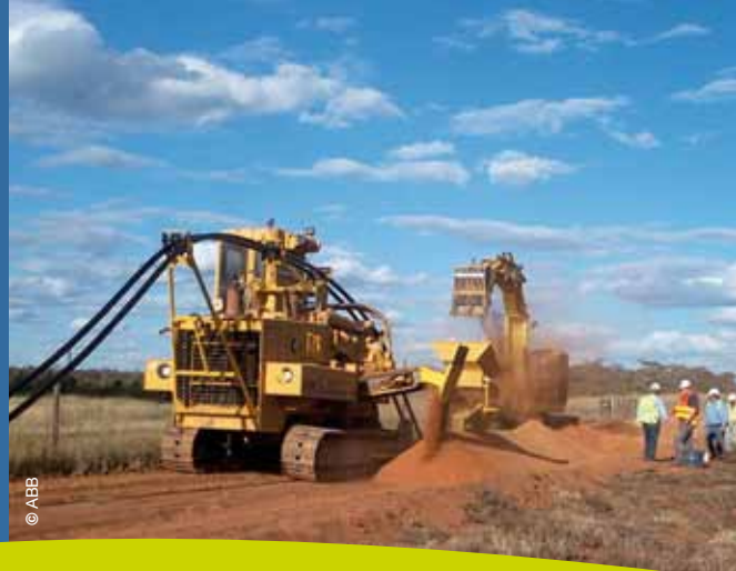
Underground cable works.
