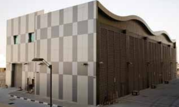
West Bay area electrification, Doha, Qatar.
