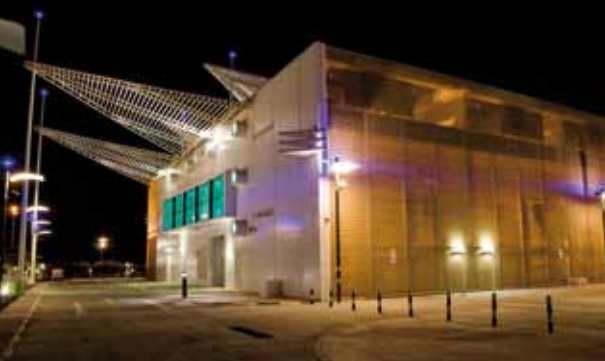
West Bay area electrification, Doha, Qatar.
