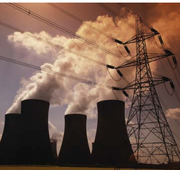
Where there are large, localised emissions, particularly from fossil fuel generation plants, there are opportunities for the capture of CO 2 .
