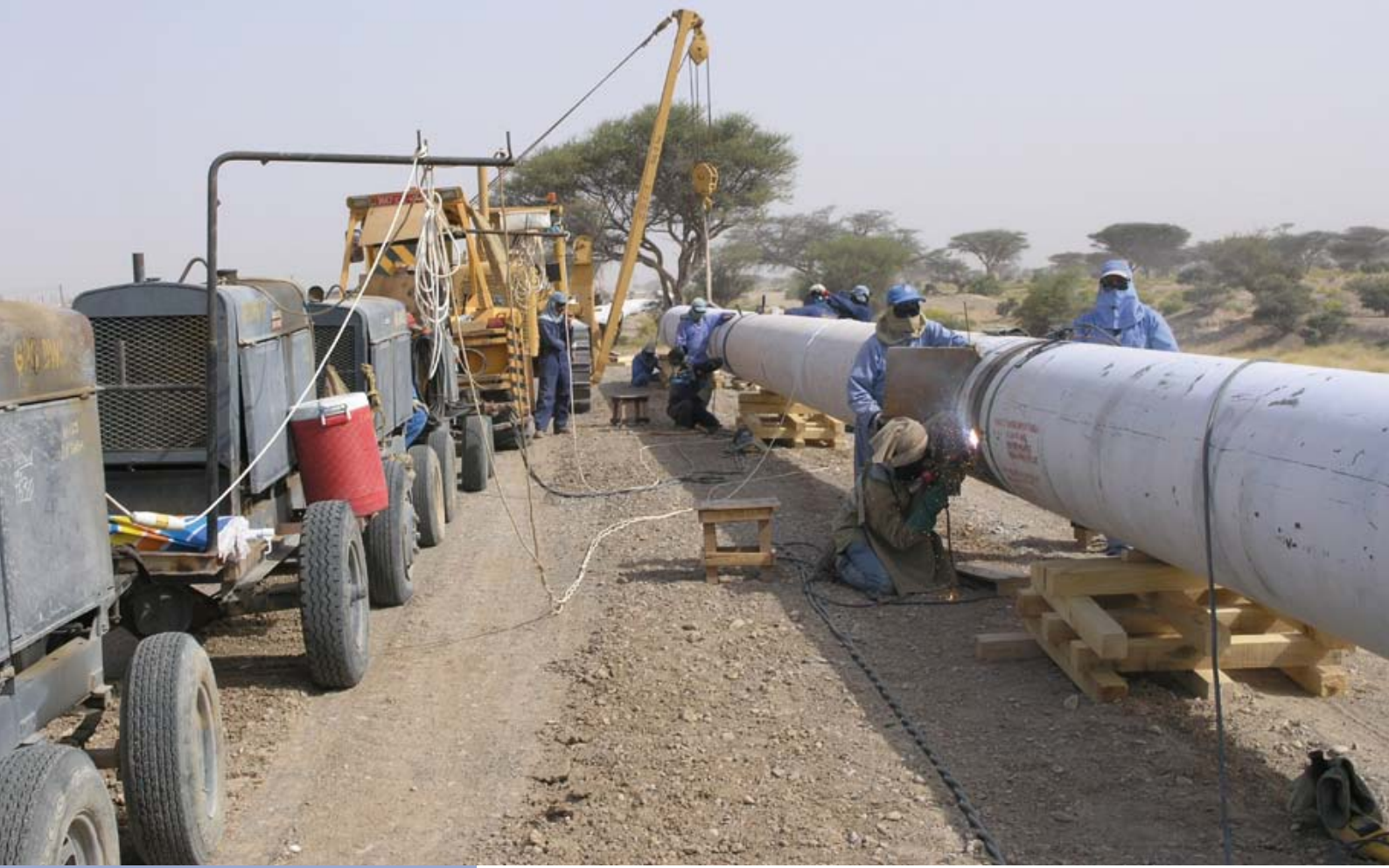
Pipeline trench construction and welding prior to trench installation – Mott MacDonald was contracted as the PMC contractor for these major works in the Middle East (above and below).
