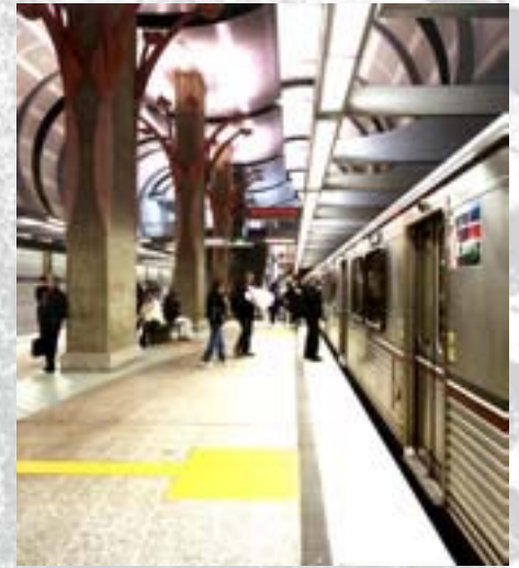
As part of a joint venture we were appointed to manage construction of the North Hollywood extension to the Los Angeles Metro Red Line
