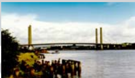
The George Street Bridge over the River Usk, the first modern cable stayed bridge in the UK, opened in 1964
