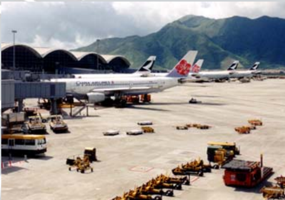
At 1.3 km long and covering over 550 000 m 2 , the Hong Kong International Airport passenger terminal with its Y-shaped concourse is the world's largest single airport building. A Mott MacDonald led consortium was responsible for project management and engineering design of the award-winning terminal
