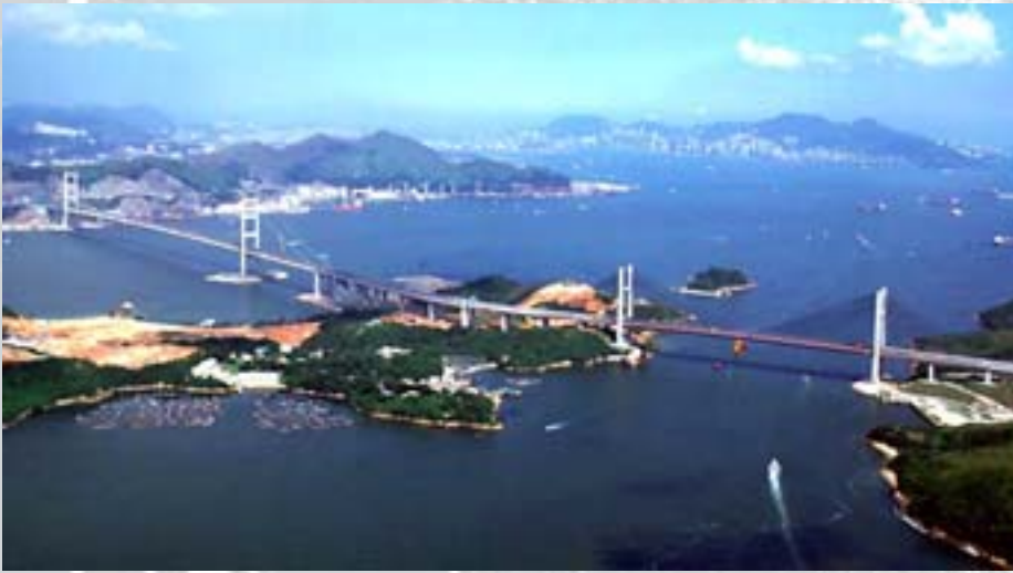
We conceived, planned, designed and managed the record-breaking Lantau Link – a strategic connection in Hong Kong's road and rail transport network
