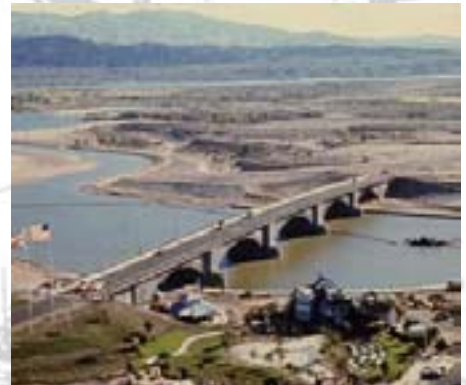
Each year an estimated 1.5 million tourists from all over the world flock to view the old granite London Bridge which we helped to construct across a man-made channel at Lake Havasu in Arizona, USA
