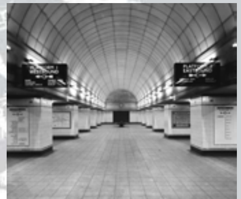
Our pioneering work on reinforced concrete tunnel linings was put to the test on the final section of the Central Line extension between Redbridge and Newbury Park. The technique was later used world-wide
