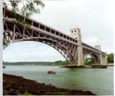
Britannia Bridge, linking Anglesey and mainland Wales, was originally designed by Robert Stephenson as a rail link. When it was damaged by fire we redesigned it as a twin deck bridge carrying both road and rail
