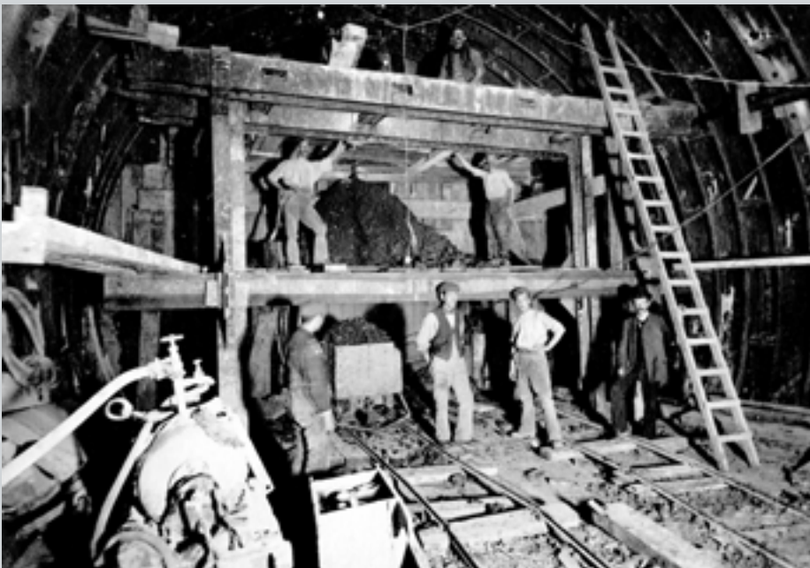
Both Basil Mott and David Hay worked on the City and South London Railway – seen here under construction at Clapham in 1898 – later to become the Northern Line
