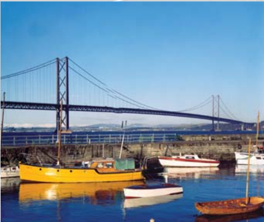
The Forth Road Bridge, Europe's longest suspension bridge when it was completed in 1964, has a centre span of some 1000 m. The scheme included nine miles of roads incorporating 14 bridges and one 180 m viaduct
