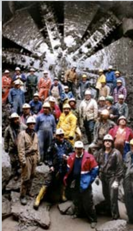
Together with Hatch Associates of Canada we designed the 1800 m long St Clair River Tunnel in Ontario, driven by a 9.52 m diameter earth pressure balance machine – at the time the largest ever used in North America
