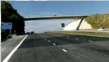
On the M3 London to Southampton motorway we designed a 24 km section between Basingstoke and Winchester featuring two river crossings
