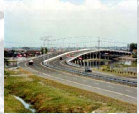
The 100 km Surabaya-Malang highway in east Java has a dual two-lane highway and 55 new bridges, including the 266 m long Surabaya River Bridge and a new crossing of the Porong River
