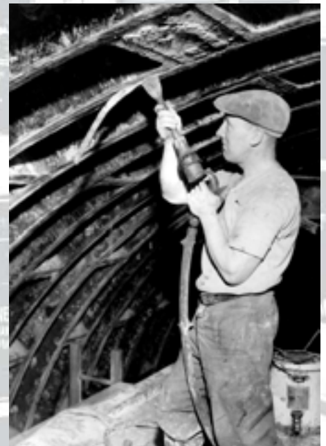
Caulking the cast iron lining of the Dartford Tunnel
