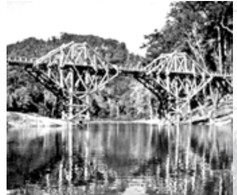
The Bridge over the River Kwai is known the world over. For the film starring William Holden, Jack Hawkins and Alec Guinness we helped design a replica bridge in Sri Lanka
