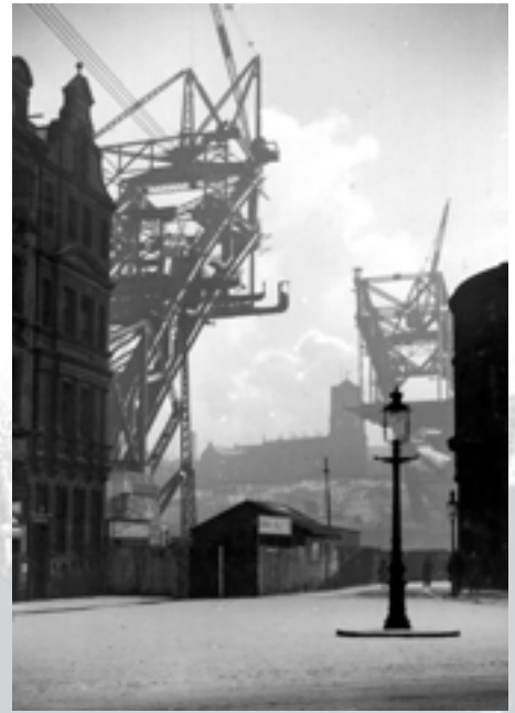
The Tyne Bridge in Newcastle, opened in 1928, was our first major project in the north east of England
